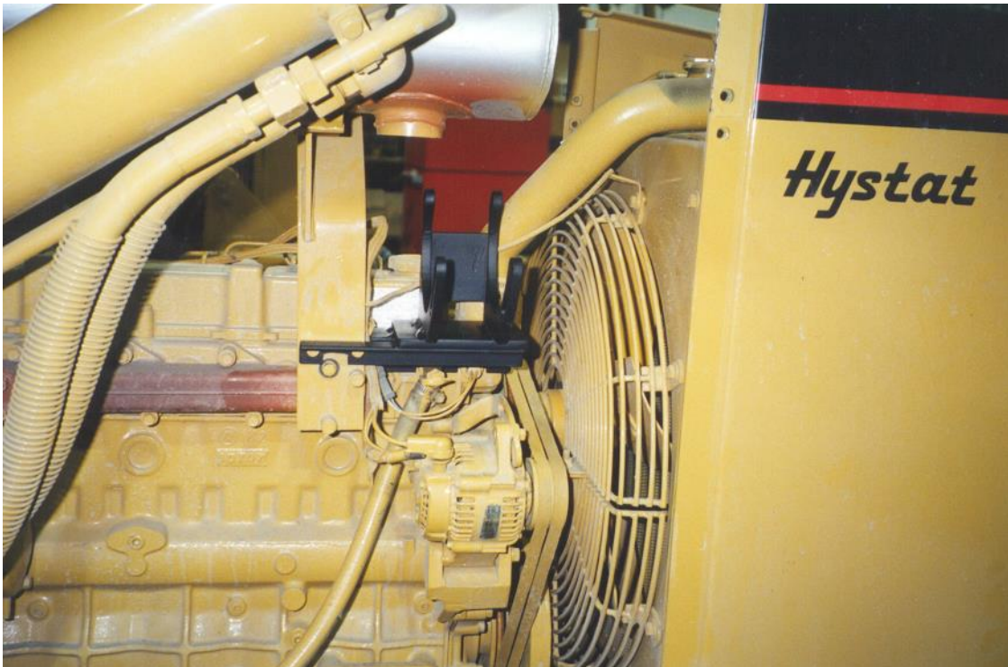
Compressor mount in place.
