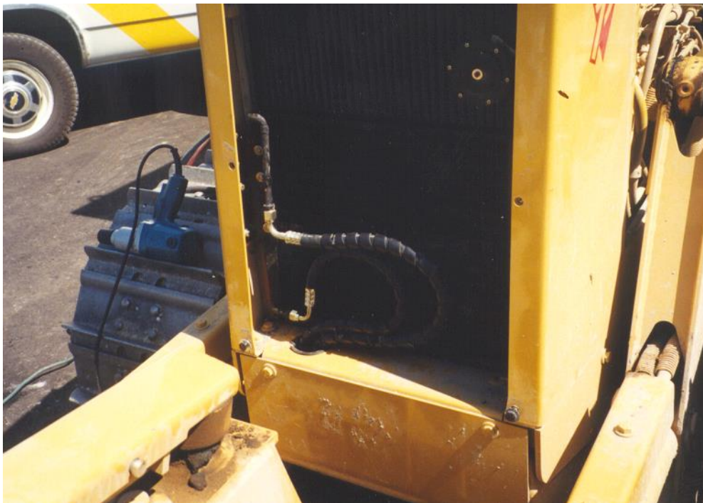
Condenser view showing hose routing.
