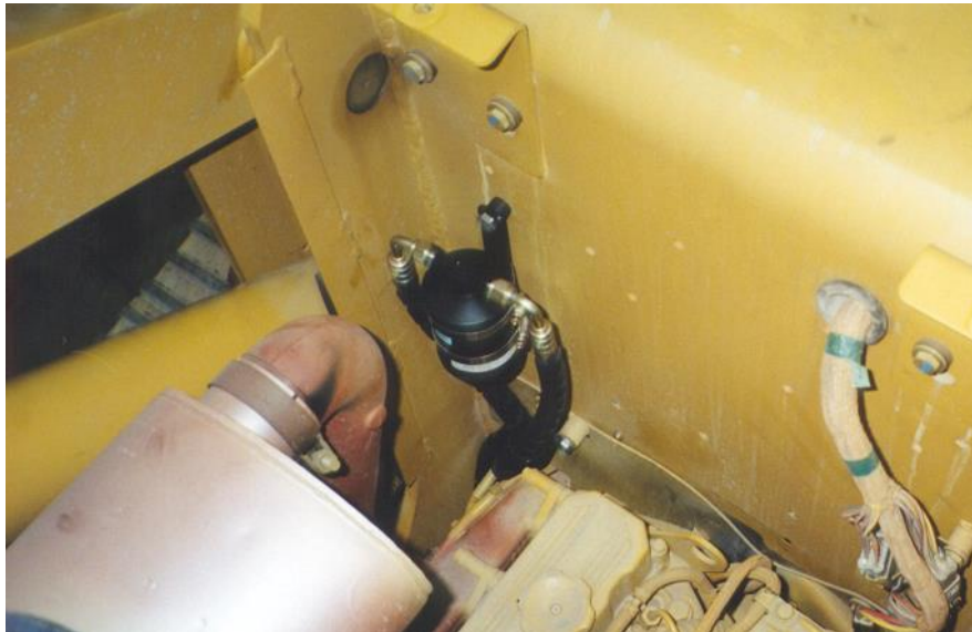
Drier in place against firewall.
